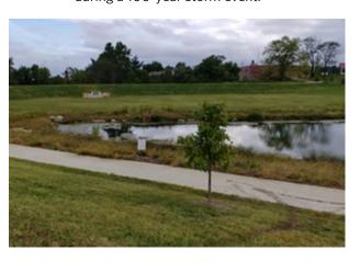
The city of Kansas City, Mo. built 150 green infrastructure installments in this Action Area to reduce the volume and frequency of overflows from the City's combined sewer system and to be in compliance with a 2010 Federal Consent Decree with the United States Environmental Protection Agency.
